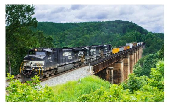
An impressive structure, this railroad bridge was built between 1915 and 1919 and is still in use today. The tallest columns are two hundred feet above the streambed.
